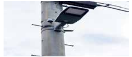
①蓄電池式防犯灯
